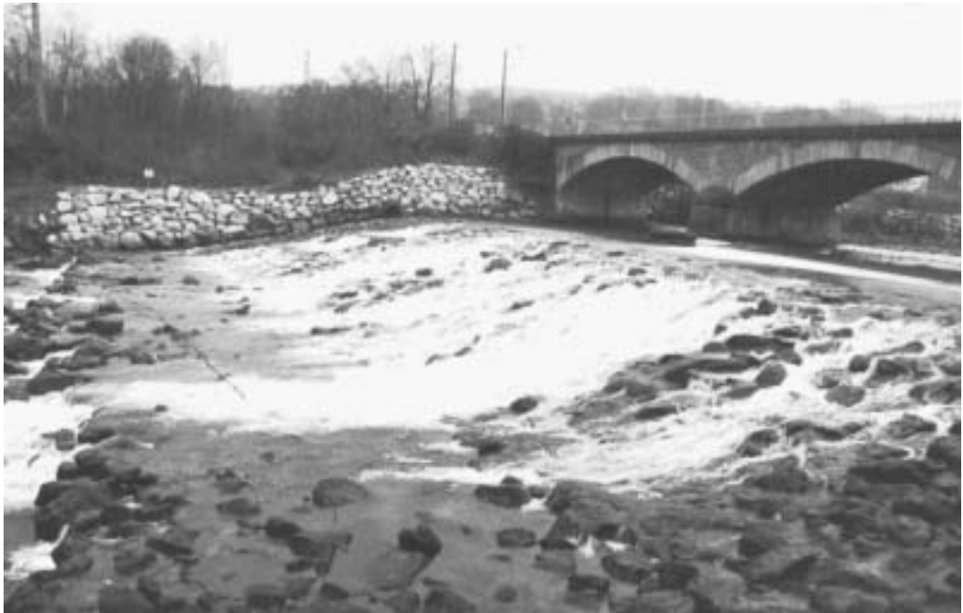
Fig. 1 - Weir at Vongy ("Le Messenger")
